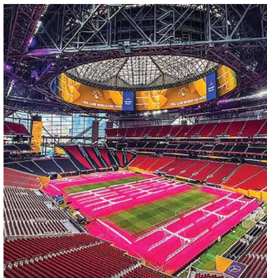
SGL LED grow lighting technology at Mercedes-Benz Stadium, Atlanta
